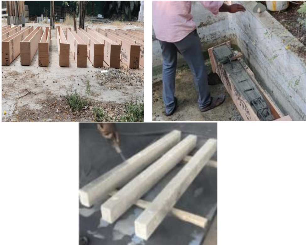
Figure 1 Casting and curing of RC beams
